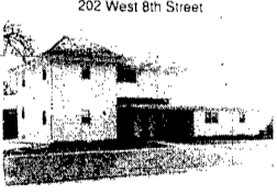
5 Unit Apartment House 100% Occupied
